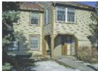
HERITAGE LANE St. Albans, 28 Homes
