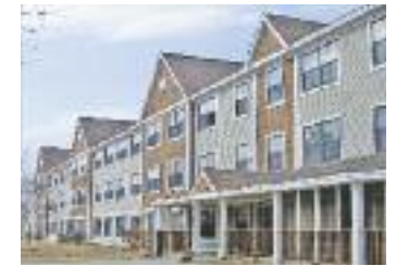
HEINEBERG SENIOR HOUSING Burlington, 82 Homes
